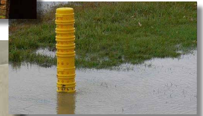
Single riser pipe attached
