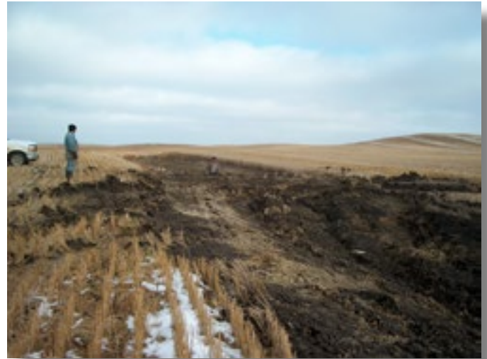
Figure 2. This photo is an example of a drainage works that was closed in response to a RFA by installing a ditch block. Respondent is now in compliance with The Water Security Agency Act .
