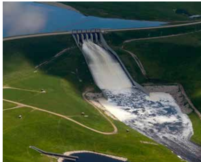
Alameda Dam spillway, Souris River flood, June 23, 2011 Photo by United States Geological Survey
